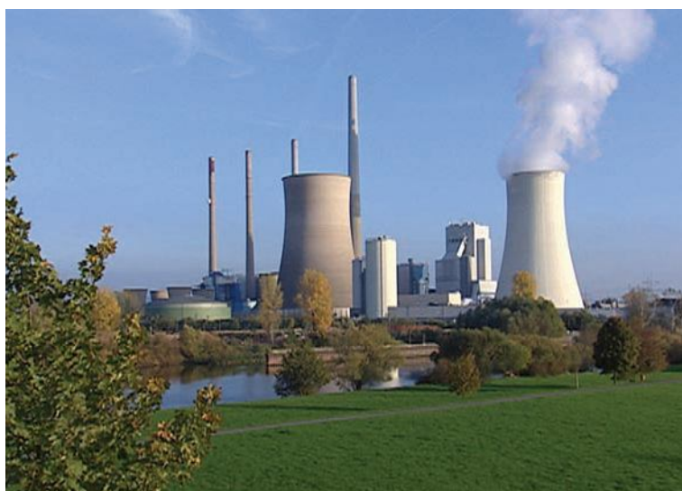
E.ON's Staudinger plant in Grosskrotzenburg near Hanau, Germany (Source: E.ON AG)
